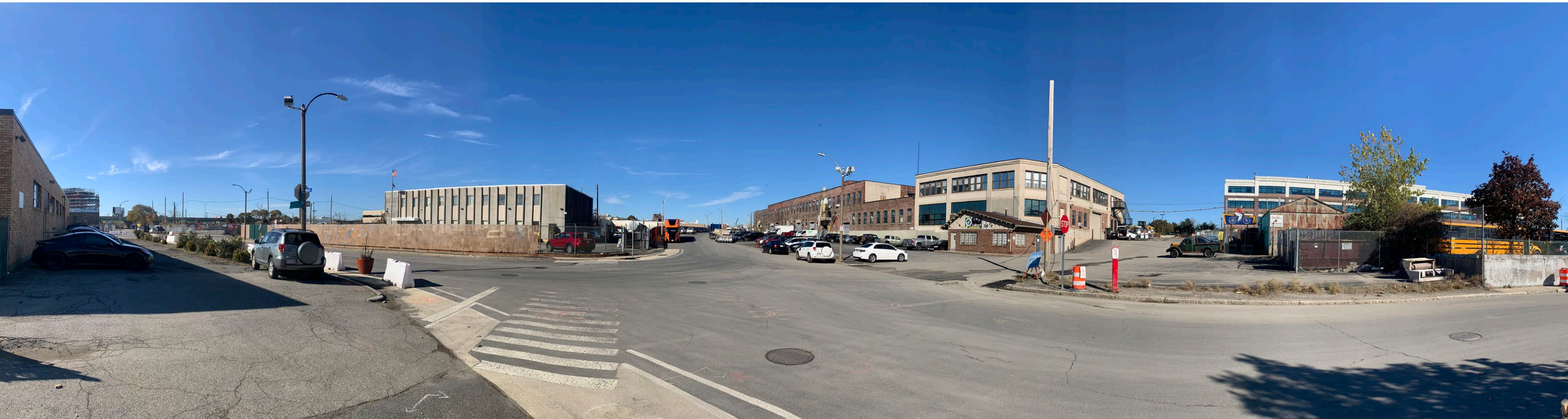
View of the current conditions of Poplar Street at its intersection with Joy/Chestnut Streets
