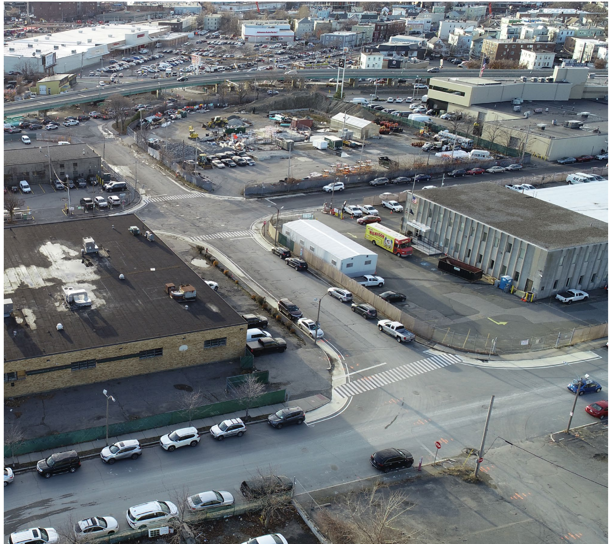
View of the current conditions of Poplar Street looking towards McGrath Highway
